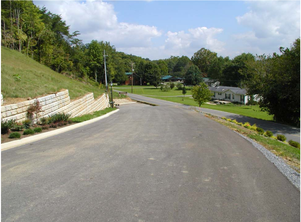
Photo 1. Photo of the Entrance Road and Retaining Wall 3 Months After the Incident.
