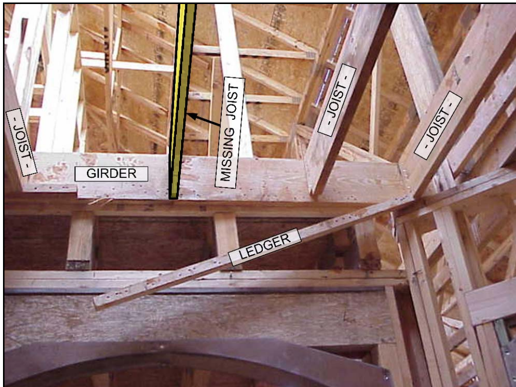
Photo 2: This photo illustrates where the ledger separated from the girder to which it was nailed and illustrates the location where the worker fell through. Note the missing joist. (Photo courtesy of NCDOL/OSH).
