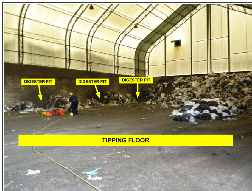
Photo 1. Photo of the tipping floor where the incident occurred showing the location of the separated materials and the pits where the waste is ram-fed into the digester tubes. (Photo courtesy of local Police Department)
