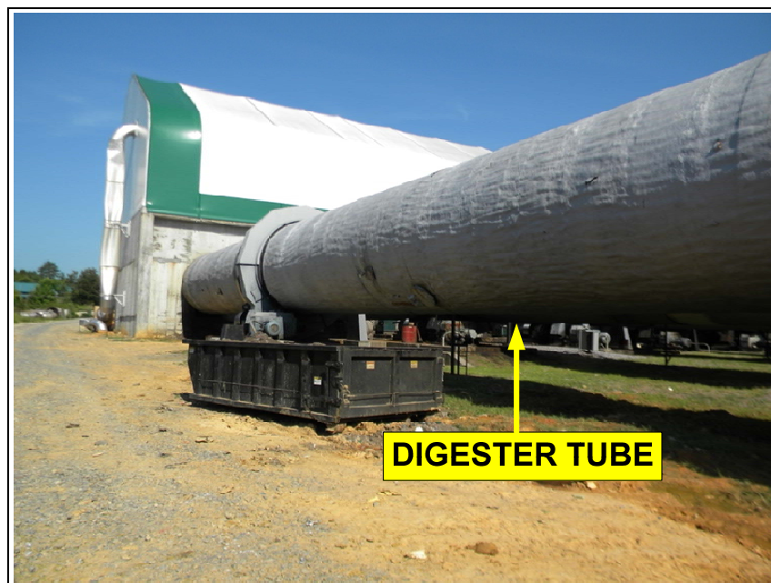
Photo 5. Photo of the digester tube extending from the tipping floor to the discharge area. (Photo courtesy of local Police Department)
