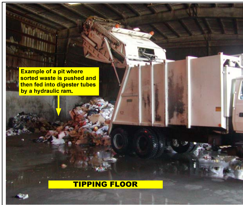
Photo 2. Photo of a truck dumping a load of solid waste onto a tipping floor. (Photo courtesy of county information on solid waste facility)
