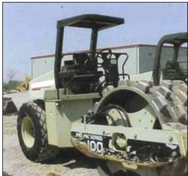
Figure 1. Pad-foot drum compactor similar to the one involved in the incident
