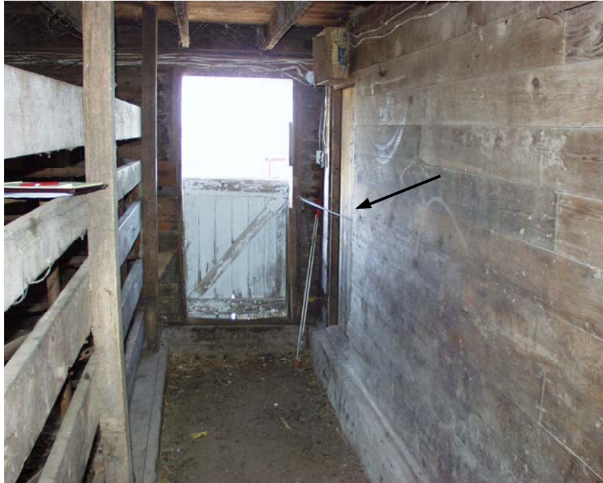
Photo #1. Looking south down walkway towards vet room door on right side. Phone was located directly inside door on right side mounted to the wall.
