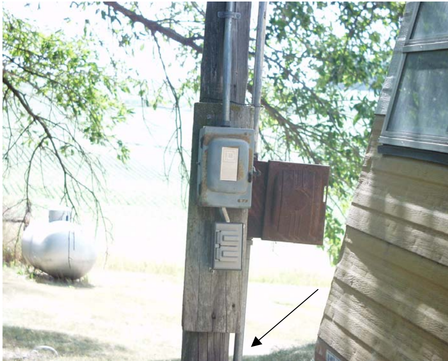
Picture #1. Pull box with conduit running to adjoining bins.
