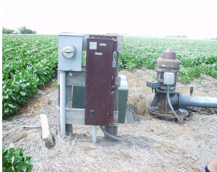
Picture #2: Commercial power source used to run well head water pump.
