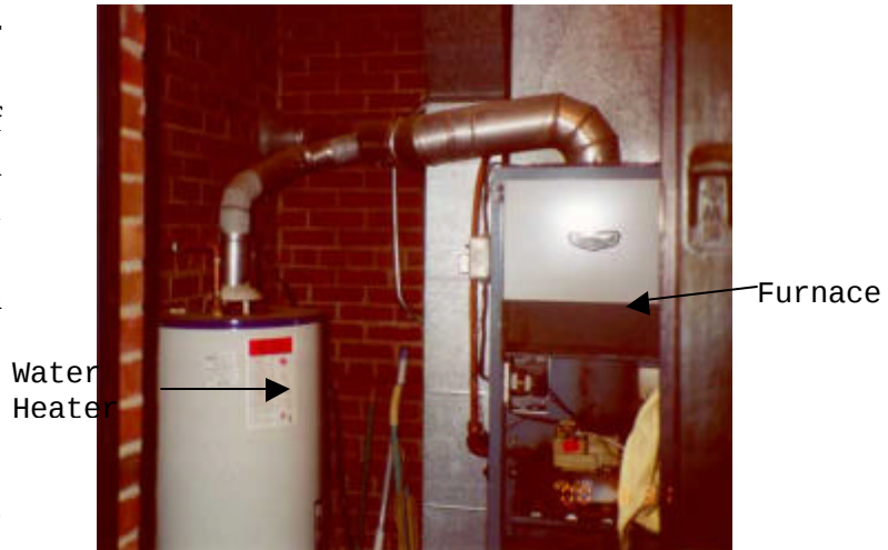
Figure 1. View of Furnace Room
