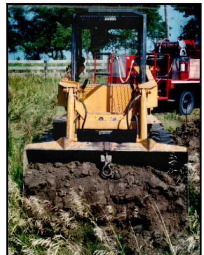
Photo 4 – Front view of loader bucket full of dirt.
