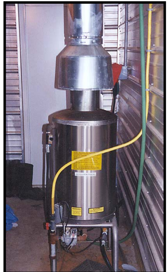
Photo 1 – Side view of LP fired heater unit.
