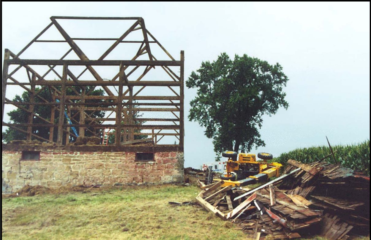
Photo 2 – View from the north side of the barn, showing the barn structure, the overturned forklift, and the broken rafter section lying next to the pile of discarded roofing.
