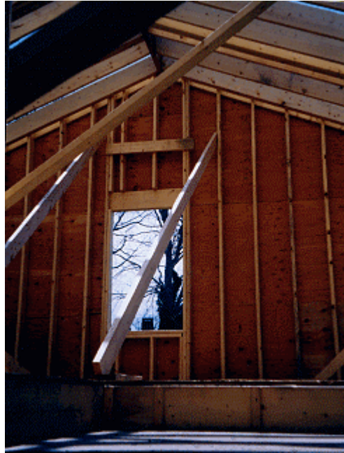
Figure 1 - Gable End 2 nd Floor Family Room
