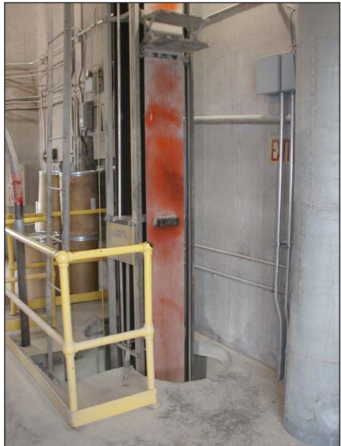
Figure 2. Manlift -- Descending Side
