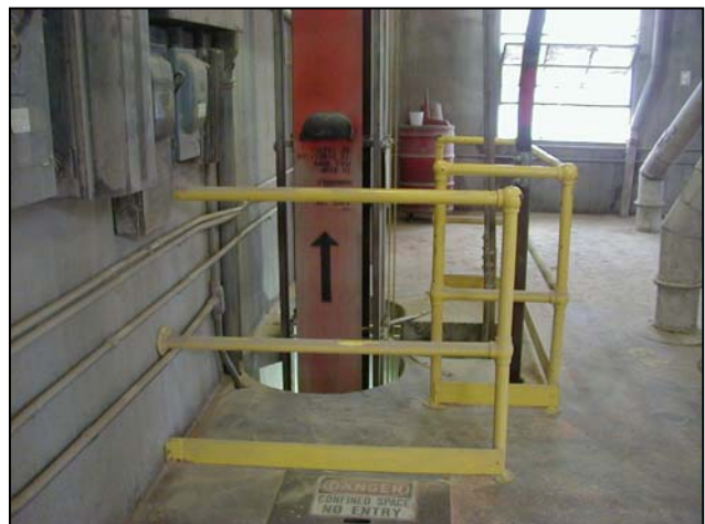
Figure 1. Manlift -- Ascending Side
