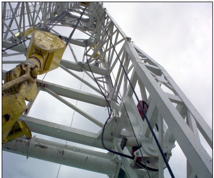
Figure 2. Oil rig cable and hoisting mechanism
