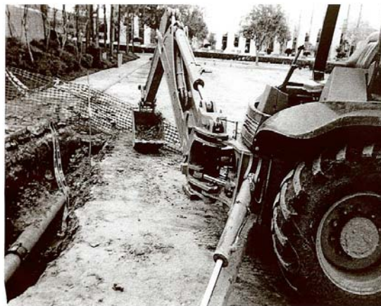
Picture 2: Bucket and Boom of Backhoe
