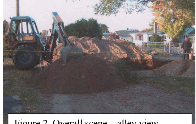
Figure 2. Overall scene – alley view
