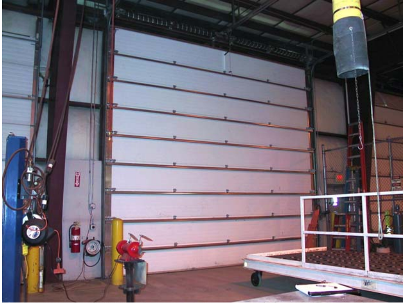
Photo 1. The overhead door that was involved in the fatal incident: a standard lift steel insulated door with six-inch lift drums. The door in the photo was adjusted and repaired by a garage door technician after the incident.
