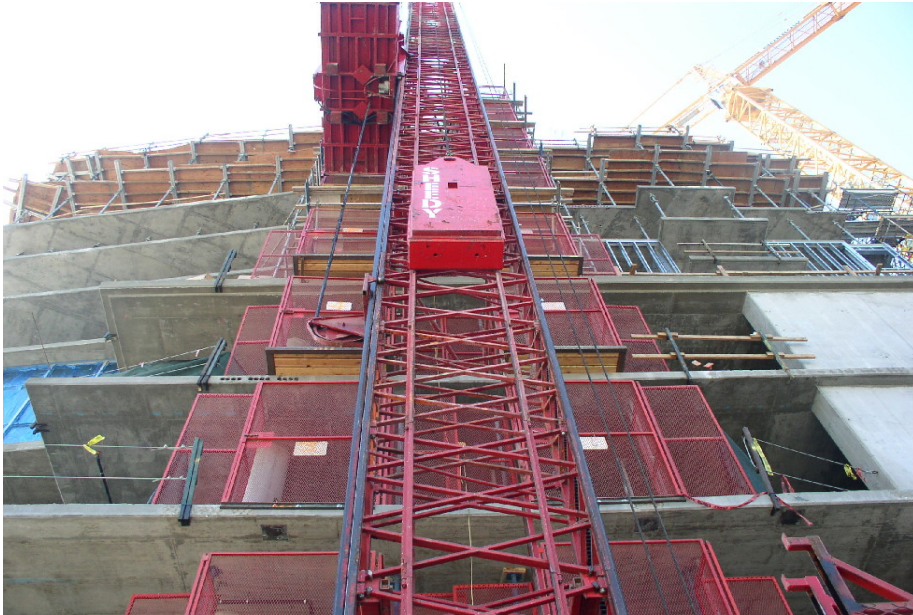
Exhibit 1. A picture of the elevator and counterweight involved in the incident.
