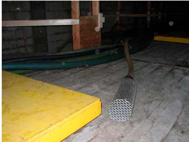
Figure 7. Brine recirculation hose with metal screen
