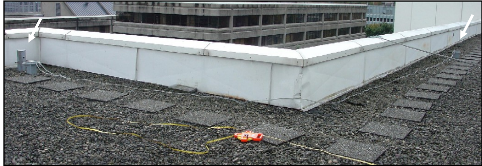
Two certified anchor points are visible here on the roof of the building where the incident occurred. The victim's anchor line was not attached to the left anchor.
