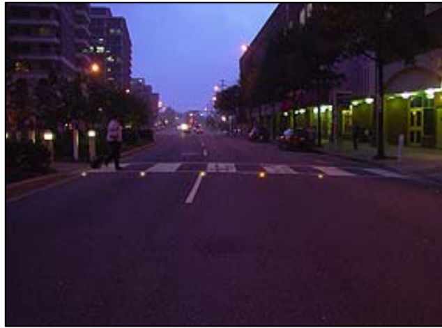
Photo 5 Example of in-road lighting system USDOT Website Photo
