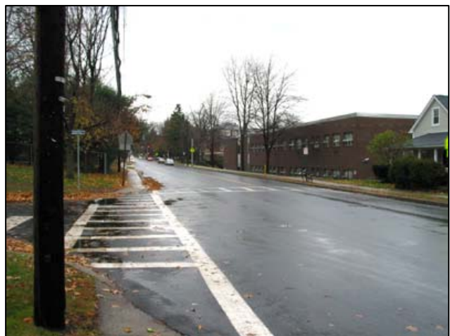
Photo 4 Photo of intersection facing north
