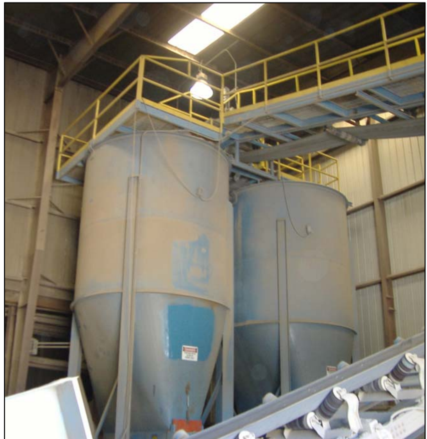
Figure 1. Silo involved in the incident
