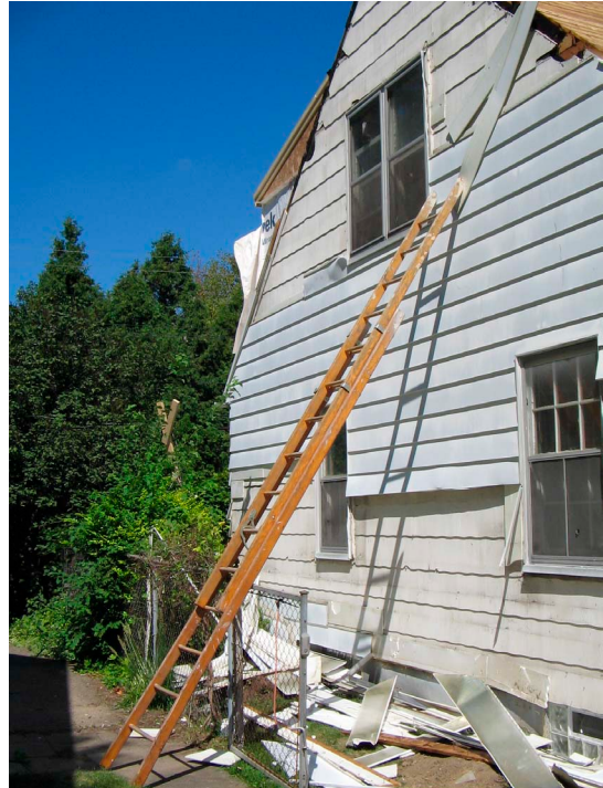
Figure 1. Siding being removed, ladder propped against fence
