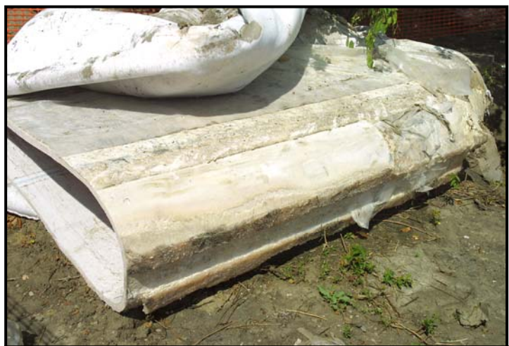
Photo 2 – Section of uncured fiberglass liner.
