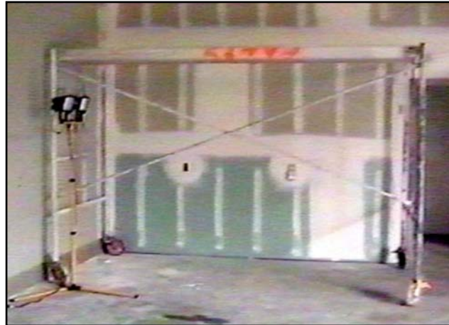
The scaffold used by the drywall installer and his lead man in this incident had only a single plank on the deck.
