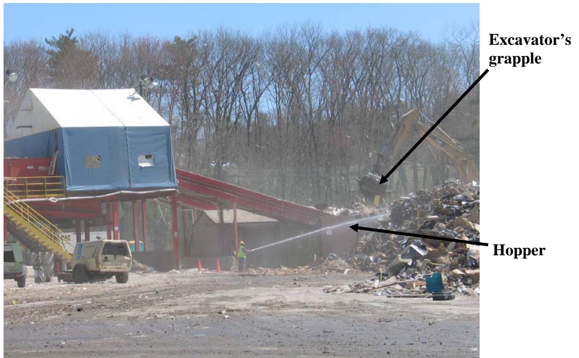
Figure 3 – Excavator with grapple loading debris into the system's hopper
