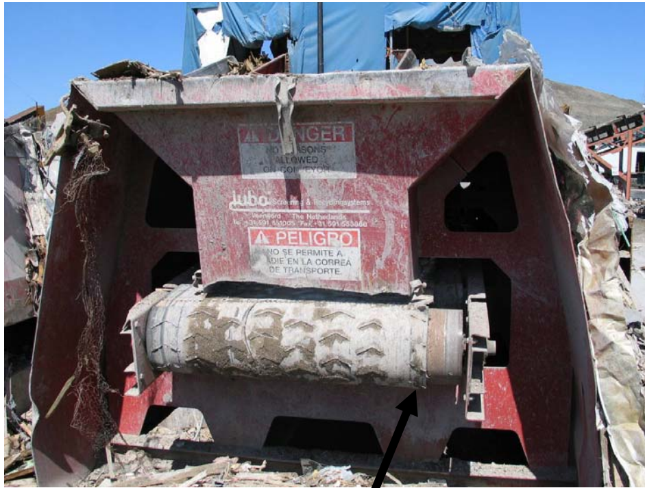
Figure 5 – Location of incident and conveyor belt
