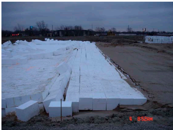
Figure 2. Ballasted edge of geofoam foundation
