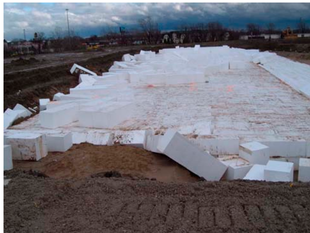
Figure 4. Incident site looking East
