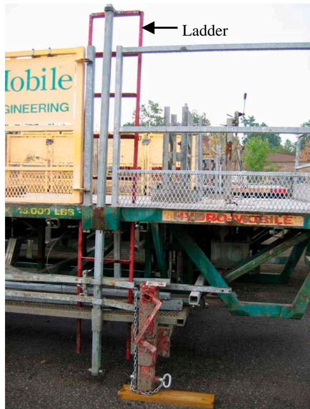
Figure 4. Ladder permanently affixed to the scaffold system.
