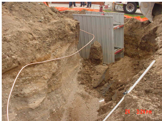
Figure 4. Position of trench box in trench during rescue operation
