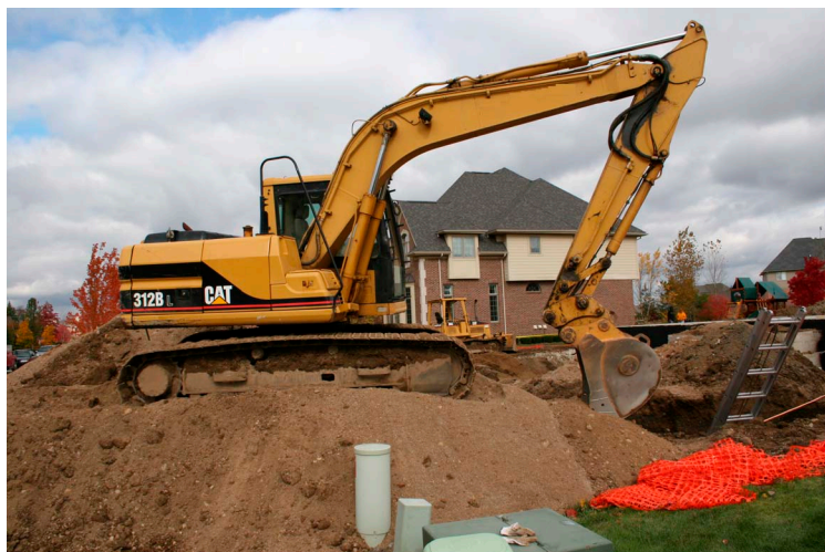
Figure 3. Position of excavator and spoils
