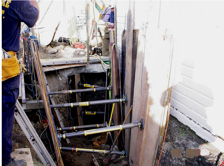
Figure 3. Shoring installation
