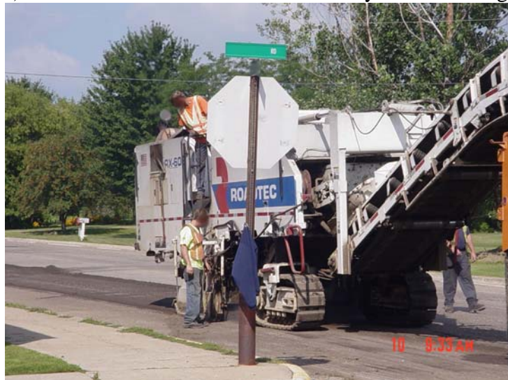
Figure 2. Typical rotomilling operation with rotomill operator and two ground men
