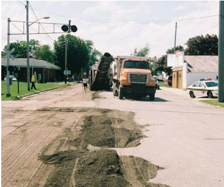
Figure 5. Position of dump truck and rotomill
