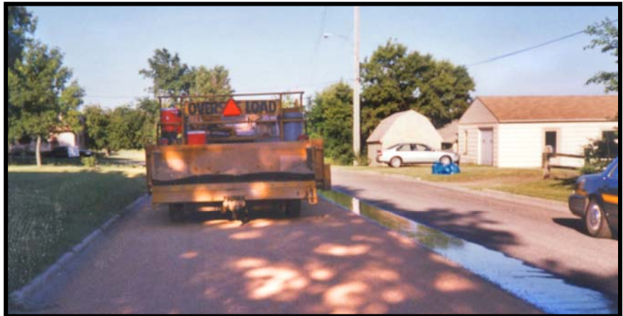
Photo 4 – Rear of the rock-chip spreading machine.
