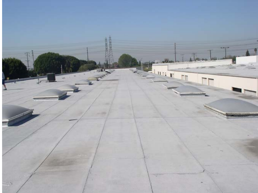
EXHIBIT 1. The roof of the building where the incident occurred.
