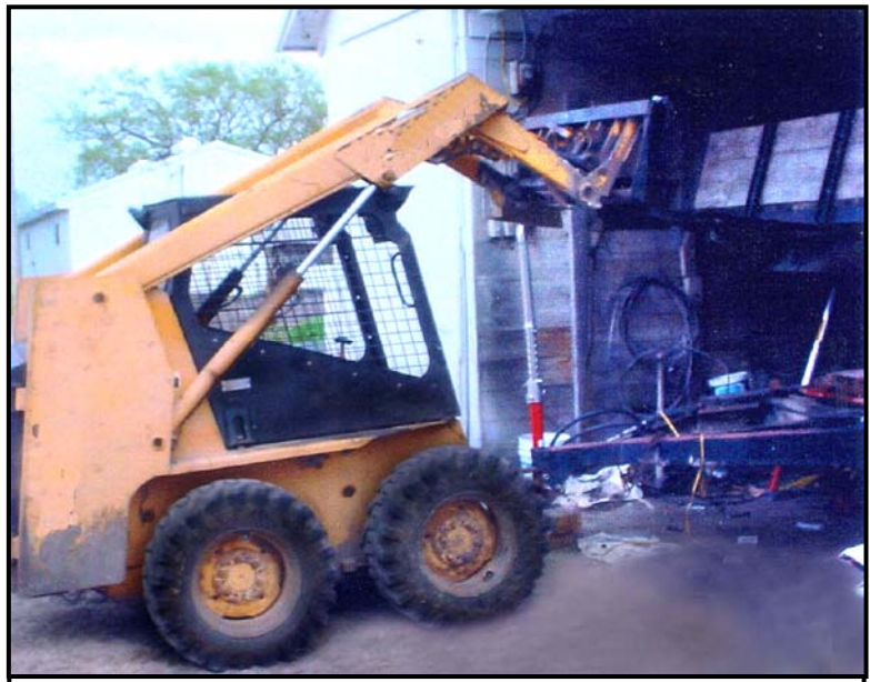
Photo 3 – Skid steer with front forks holding up the front edge of the trailer box. Also shown are the telescoping supports used by the EMS crew to secure the skid steer lift arms and trailer box.
