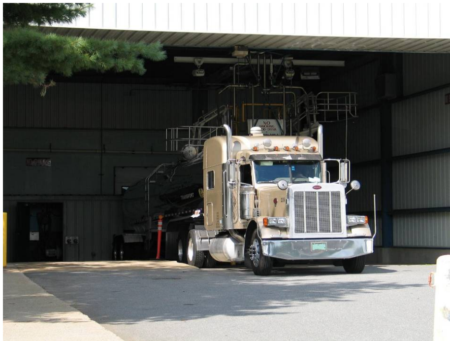
Figure 3 – Tanker truck positioned next to the platform system with a gangway lowered onto the truck's tank.
