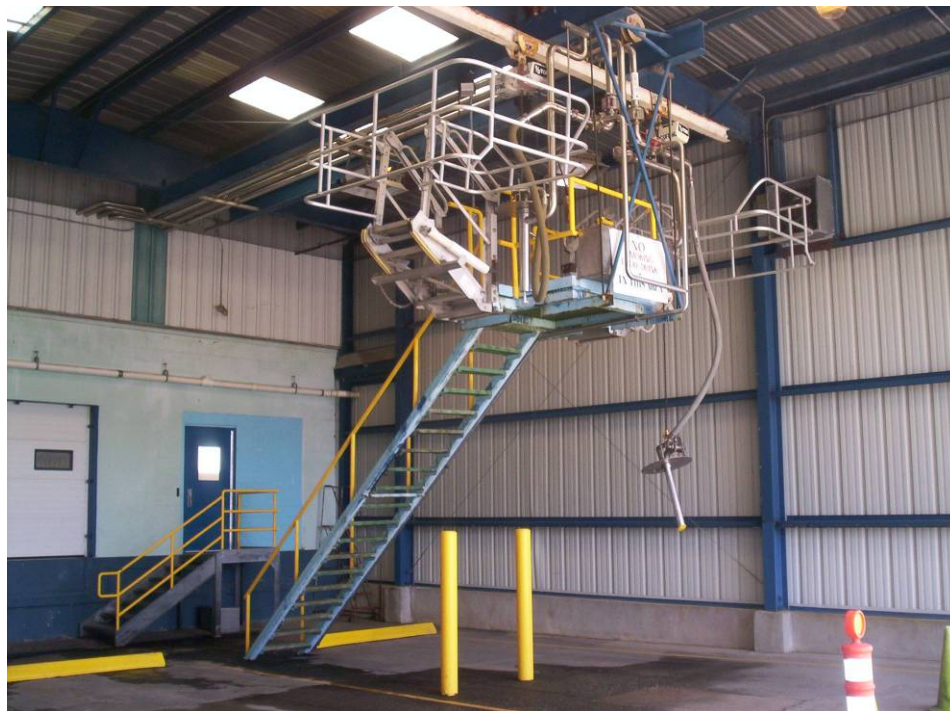
Figure 1 – Pump hose platform system.
