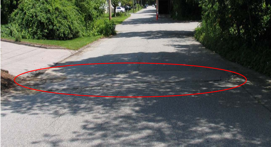
Figure 2 – Location of the incident. Roadway depression is circled in red.
