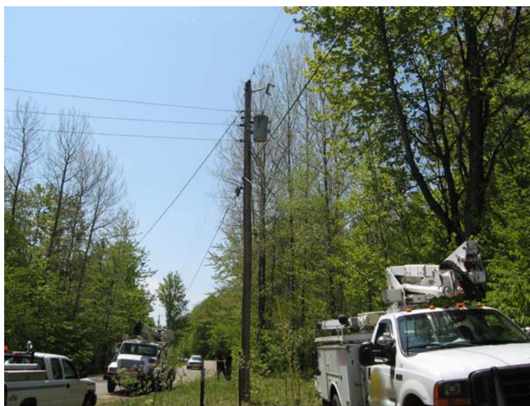
Figure 2. Location of bucket truck near guy wire, looking south
