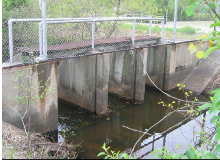
Figure 1. Upstream side of water level control structure looking east
