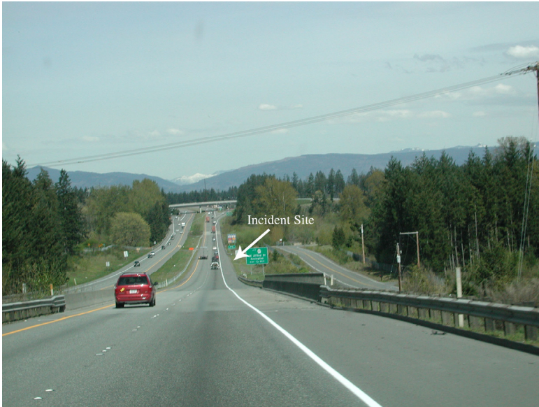
Photo 1: The view traveling down the highway east toward the incident site. The incident occurred at the bottom of the hill on the right shoulder.
