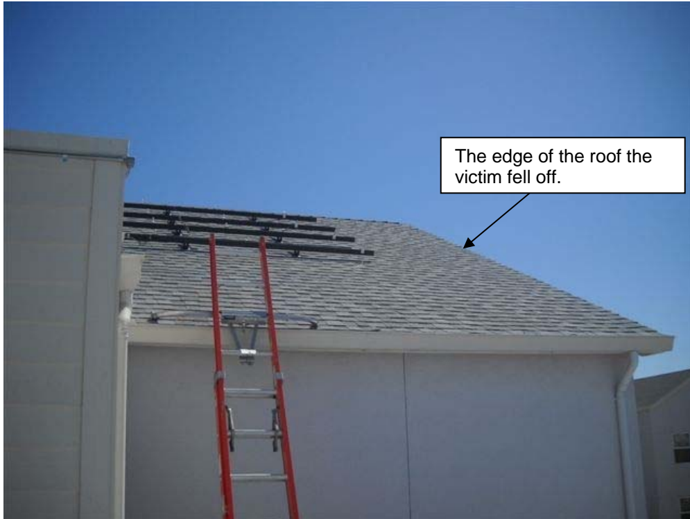
Exhibit 1. The roof edge the victim fell from.
