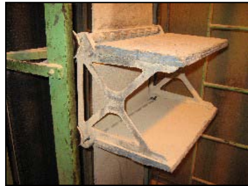
A close-up view of a platform step on the manlift shows the metal framework on the left and emergency ladder on the right.
