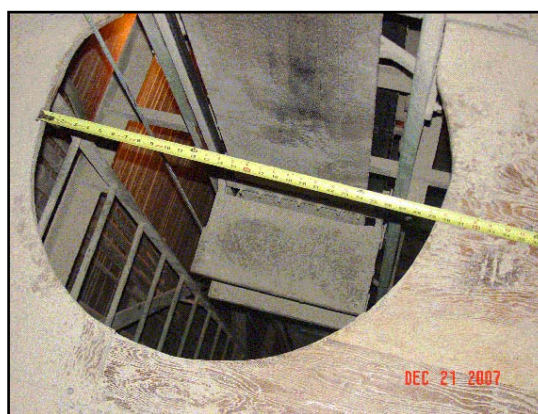
The victim fell through this manlift shaft opening. A platform step is shown on the lift belt, and the fixed ladder and stop cord at left.
