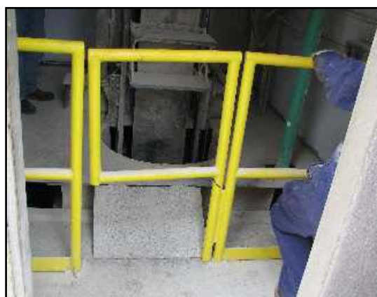
A gate guarded the manlift floor openings. At one opening, a raised plywood floor was spongy when walked upon, reducing secure footing.
