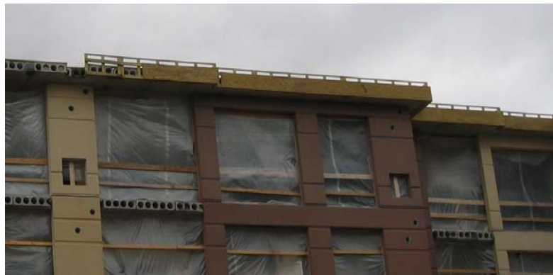
Figure 6. Example of parapet work construction
