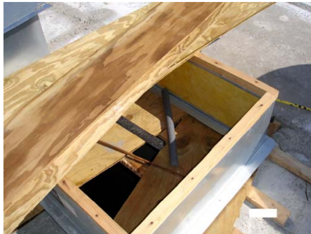
Figure 4. Chase A exhaust fan hole with 2x4 lumber and plywood boards as cover
