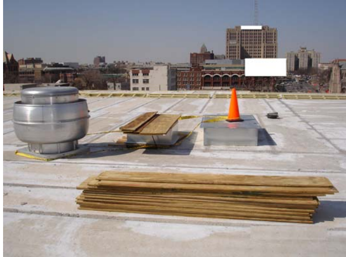
Figure 7. Make-up air roof curb with orange pylon, exhaust fan roof curb with plywood, looking north on roof
