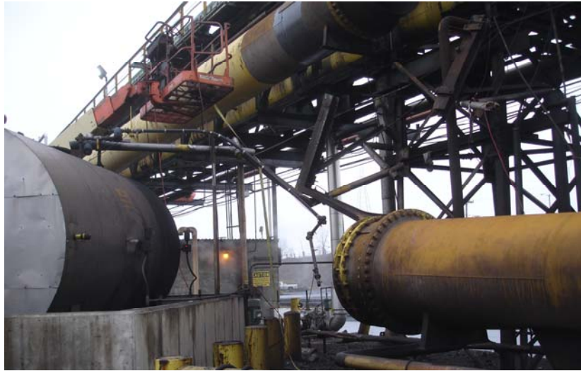
Figure 1. Incident Scene. 54-inch pipeline blown apart, area where patch repair occurred, and man lift used to elevate workers to pipeline repair area
