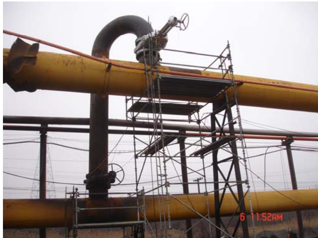
Figure 2. Example of bypass piping
