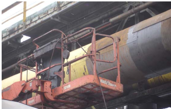
Figure 5. Gasketed steel cladding patches and man lift
