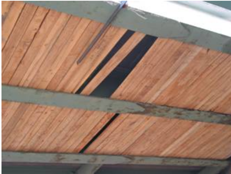
Figure 1. Example of shifting bridge deck “catch” platform wooden planks (view from ground).
