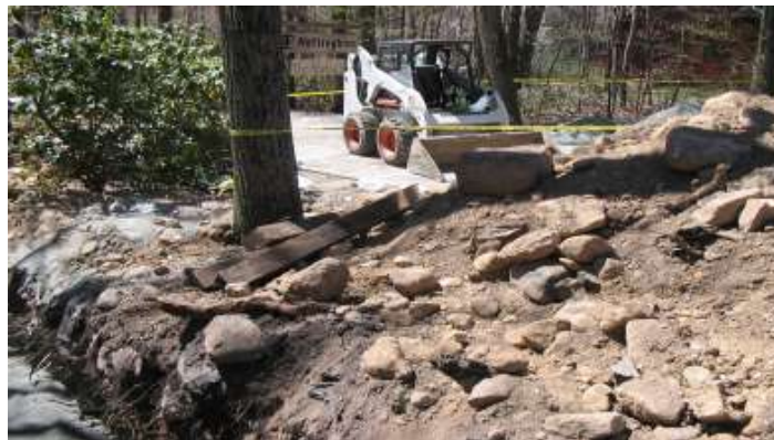
Figure 2: View of the west wall of the excavation south of the “T.” Note the boulders and loose rock/dirt on the excavation face as well as the location of the spoils pile within 2 feet of the edge of the trench. (courtesy of OSHA)
