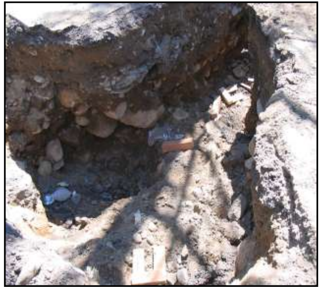
Figure 4: Area of trench collapse Note the large boulders hanging from the than excavation faces and undermined areas on the edge of the trench (courtesy of OSHA)
