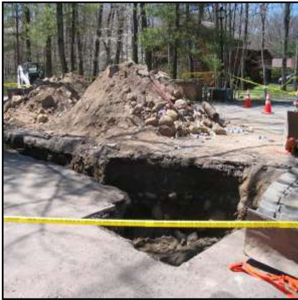
Figure 3: Location of collapse. Note spoils piles and equipment located less 2 feet from the edge of the trench (courtesy of OSHA)
