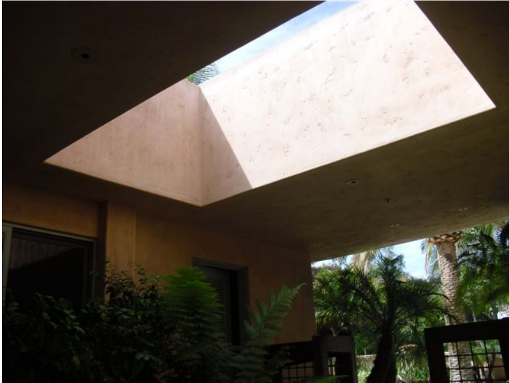
Exhibit 5 - The roof opening as seen from below.
