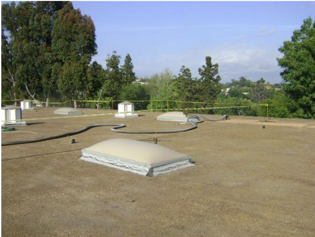
Exhibit 2. The work area on the roof.
