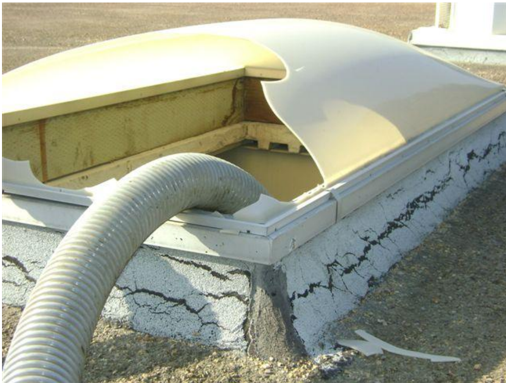
Exhibit 5. The base of the skylight.
