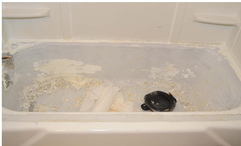
Exhibit 5: Bathtub where technician was found
