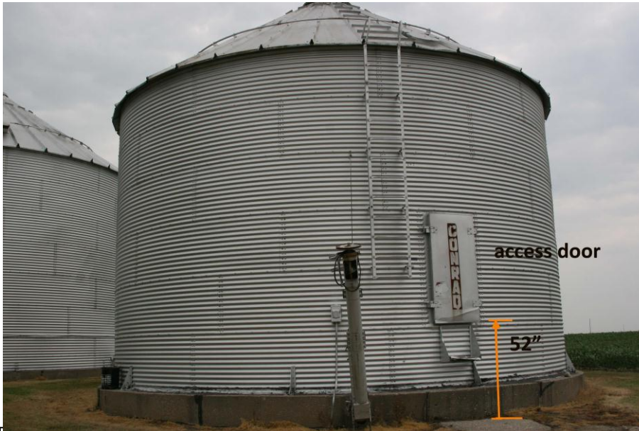
Exhibit 1: Grain bin where engulfment occurred
