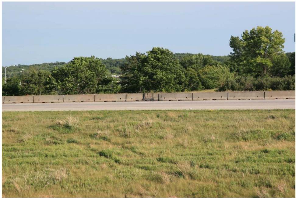
Exhibit 2. Concrete median of F-shape barriers at site
